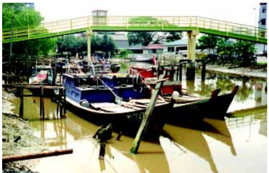
Boatyards and landing centres in Sri Lanka (top and centre) and Thailand (below) are sometimes deficient in trained manpower and adherence to safety regulations.
