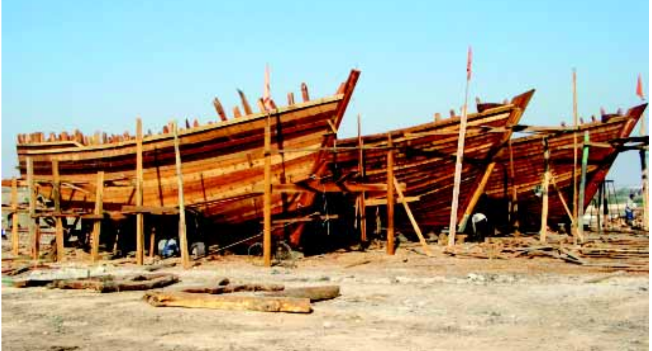
Wooden boats under construction in India
