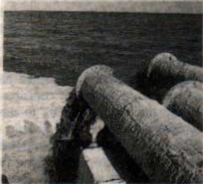
Here carry the ash slurry from the Tamil Nadu power plant only to be discharged into the sea. The slurry is a thick, black, sticky substance that is highly polluting. It is a major source of pollution in the Bay of Bengal.
