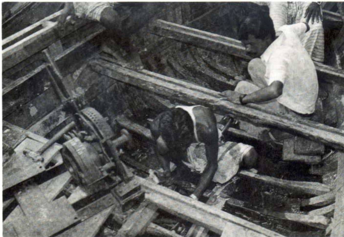
Installing an engine in a chandi boat.
