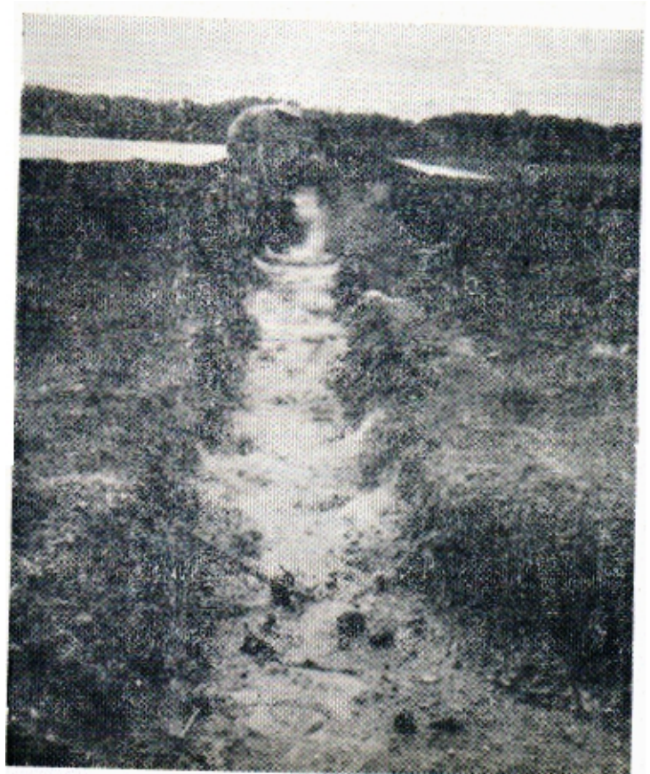
Applying lime to the soil dyke to reduce acid sulphate content of the soil.
