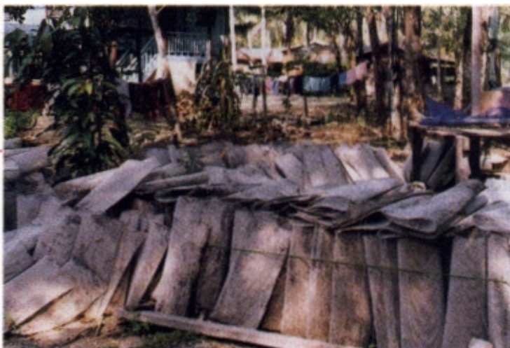
Netlon cylinders coated with cement-lime dip.
