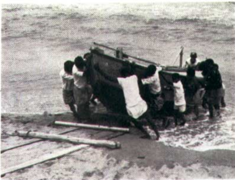
Planks and rollers placed beneath IND-10. Note steepness of the beach.
