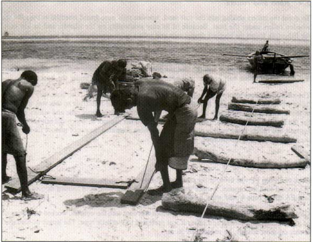
Wooden rails and sleepers are arranged preparatory to hauling ashore a dhoni
