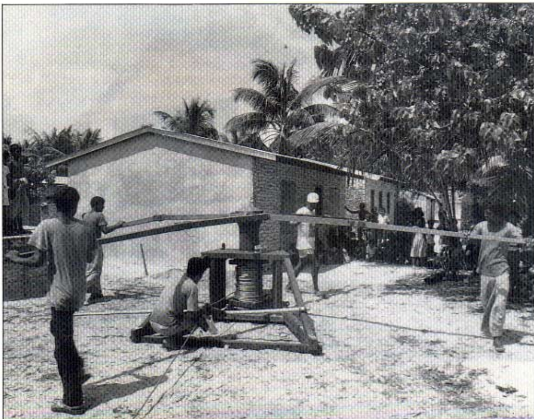
The steel wire gets wound on the wooden winch as the hauling operation gets underway
