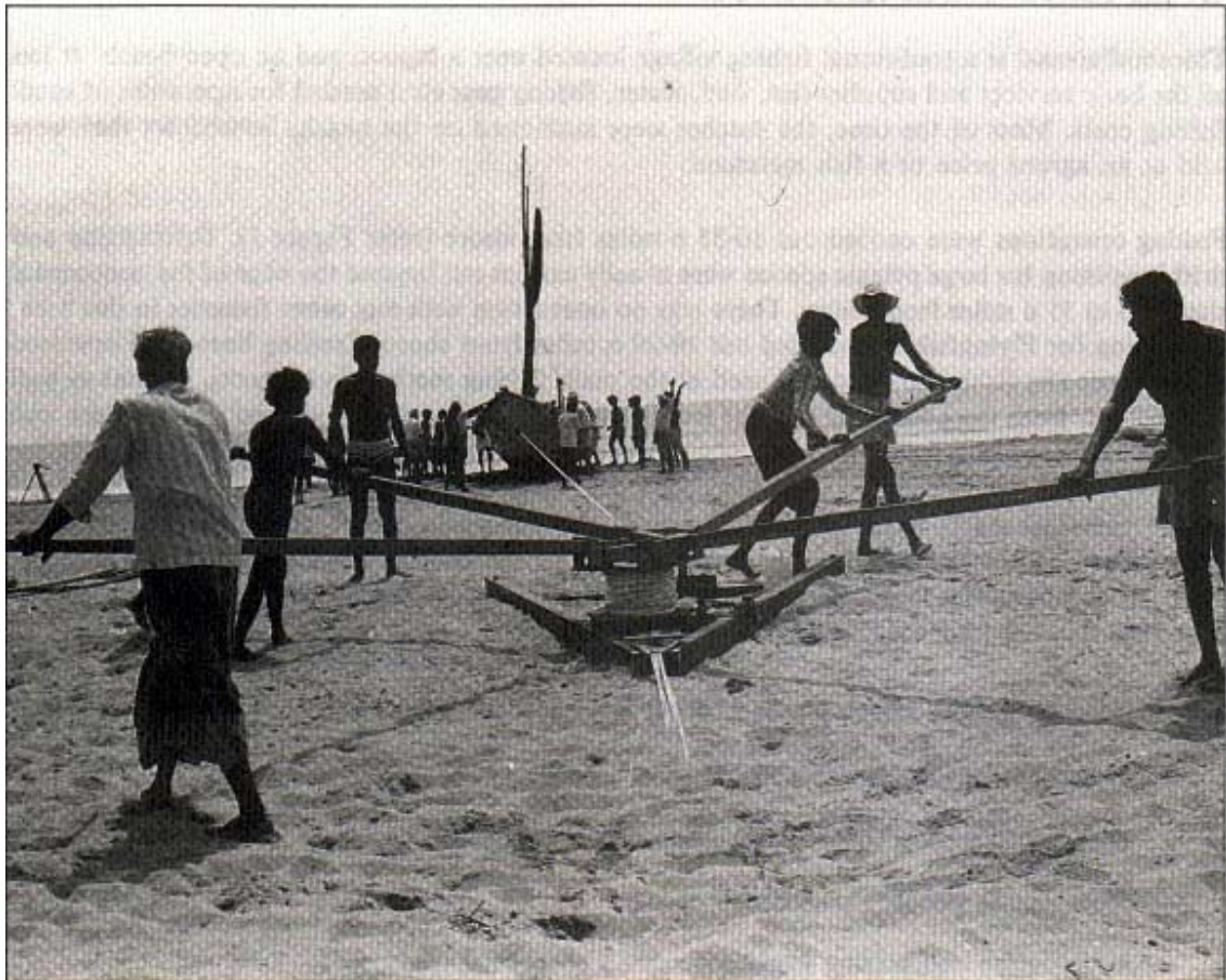
Hauling the BLC on to the beach (below) in Thirumullaivasal with a steel winch (above)
