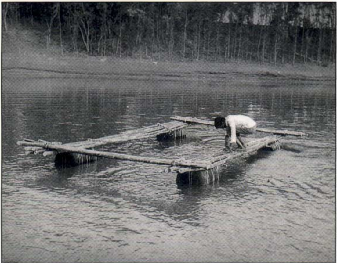
Checking the rigidity of the bamboo frame
