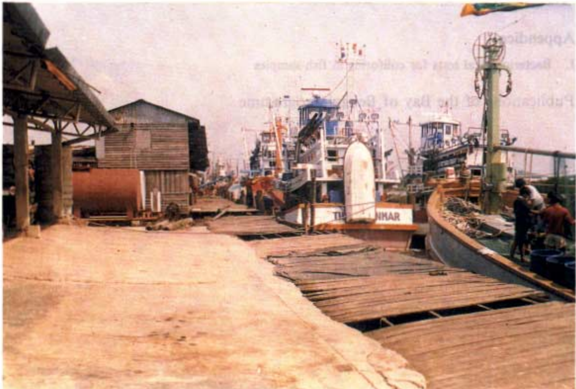
Typical private pier – Phuket
