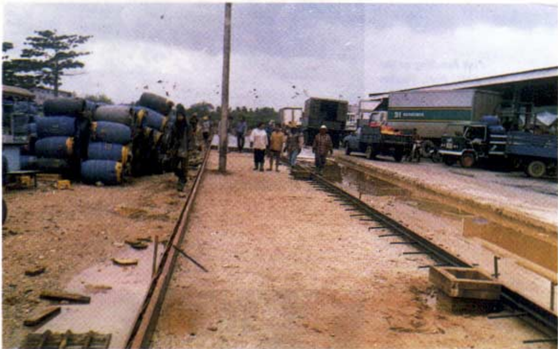
Improvement of the access road to FMO Port, Phuket
